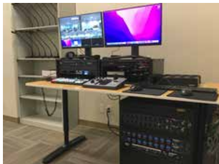
Finished MYPA Install
